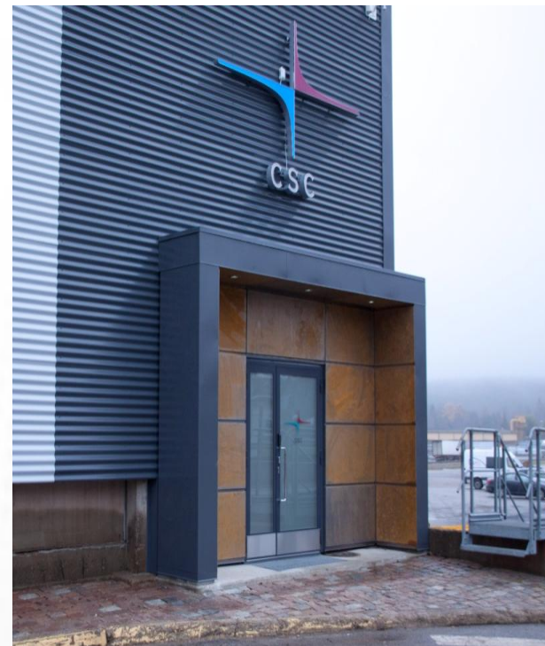
Data Center CSC Kajaani is located in the Renforsin Ranta Business Park.
