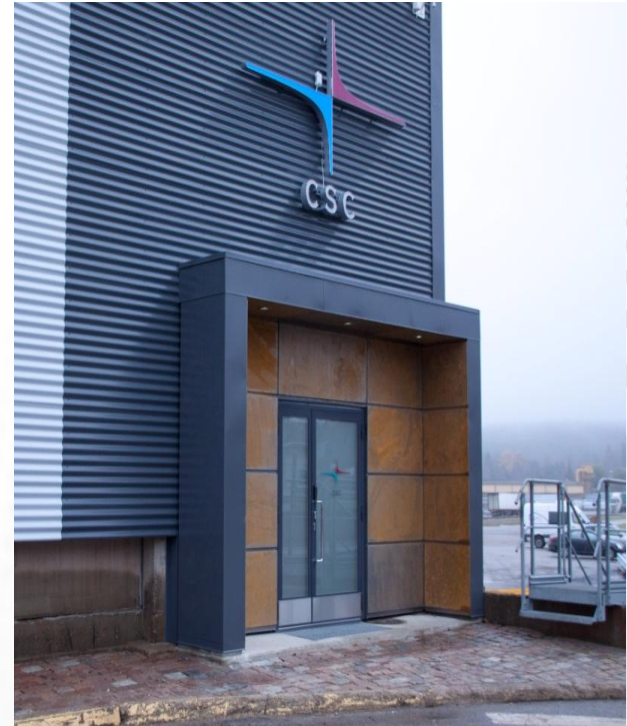
Data Center CSC Kajaani is located in the Renforsin Ranta Business Park.
